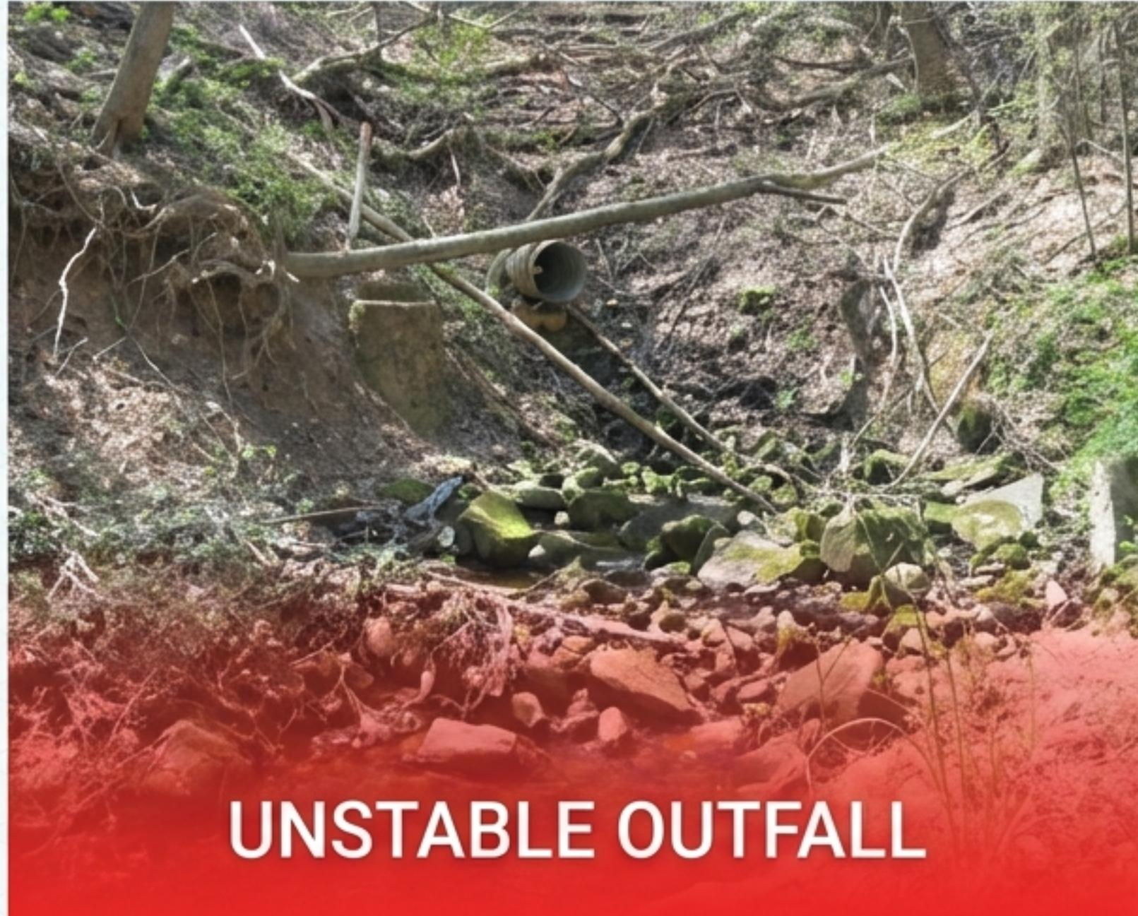
**Definition:** Localized erosion of the stream bank or bottom caused by high-velocity discharge.
