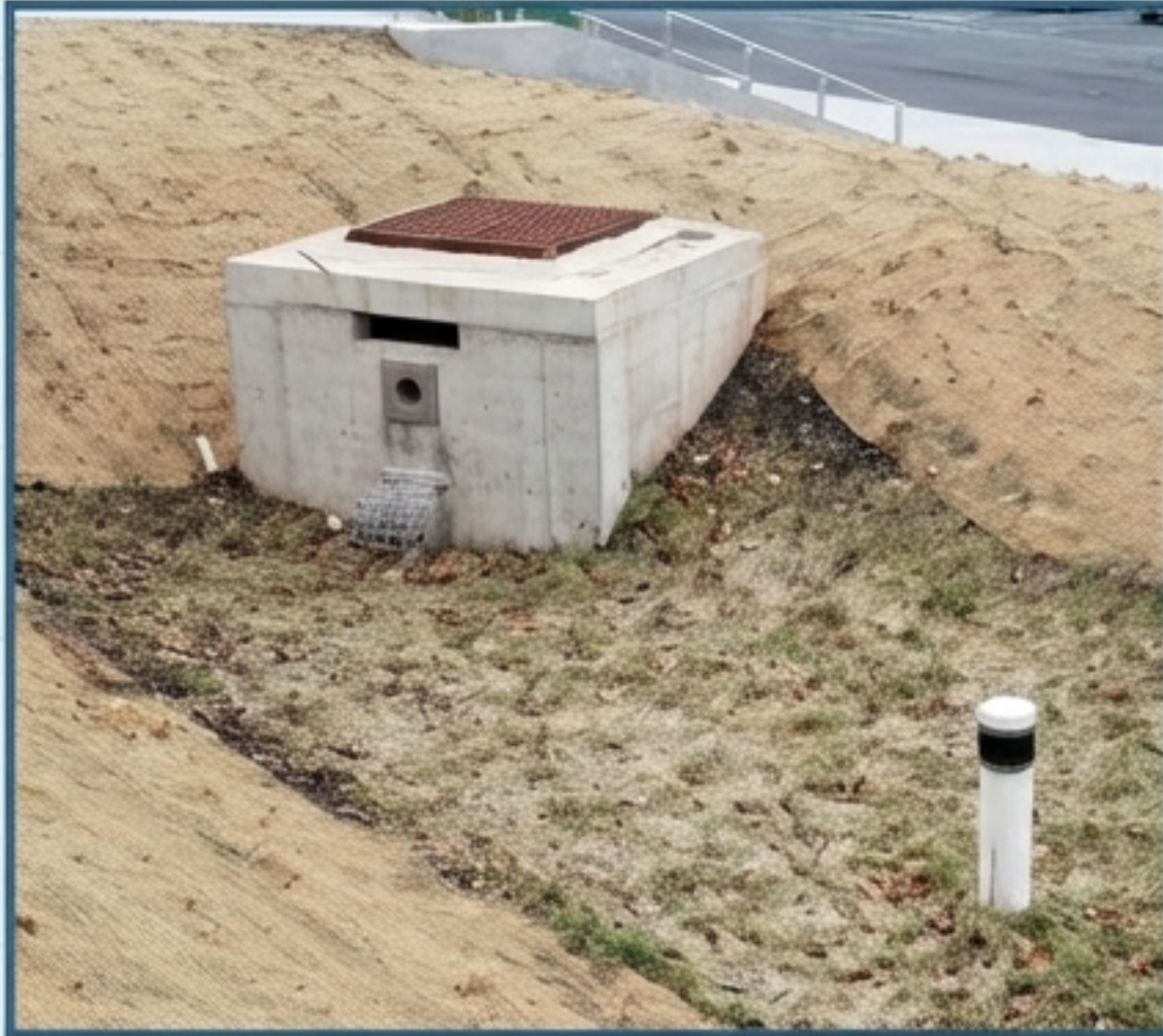
Concrete Outlet Structure with Trash Rack
