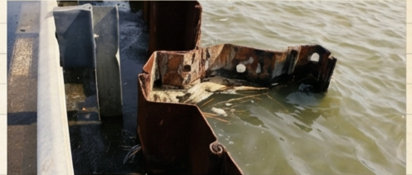
Structural Corrosion
