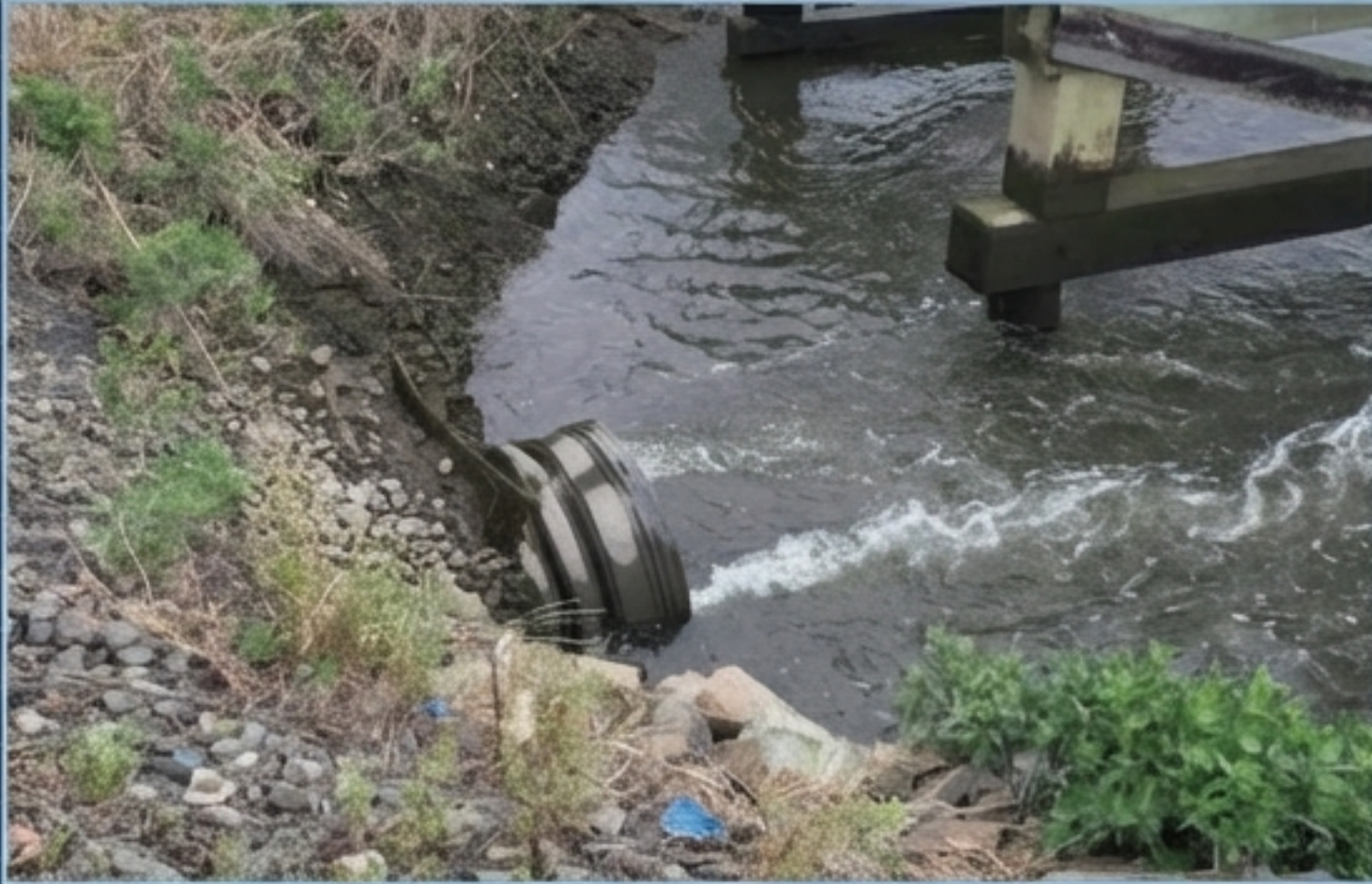
Undersized Culvert
