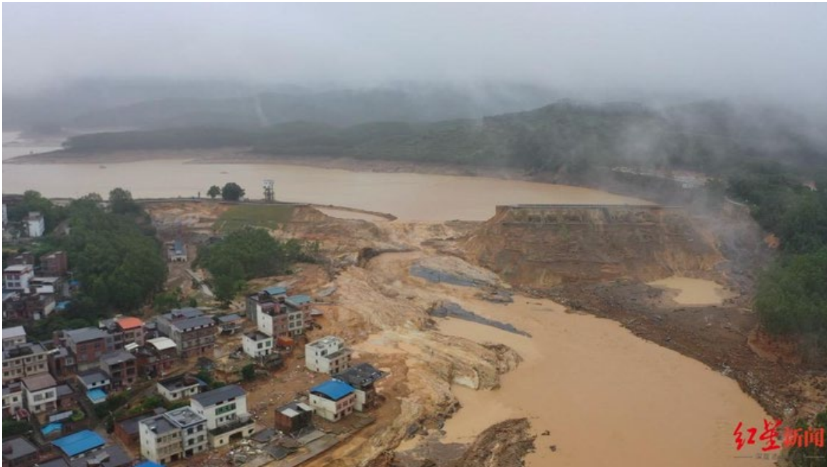
Figure 2. Aerial View of the Dam Breach and Near-Dam Downstream Area after the Liulan Reservoir Failure. The image shows the large breach, sediment-laden outflow, and affected near-dam downstream area. It documents the overall post-event scene but cannot by itself establish the initial breach location, the precise sequence of overtopping and local breaching, peak discharge, or the specific failure mechanism. Image source: Red Star News, “The Critical 12 Hours before and after the Liulan Reservoir Breach: Those Trapped and Their Rescuers,” July 11, 2026.
