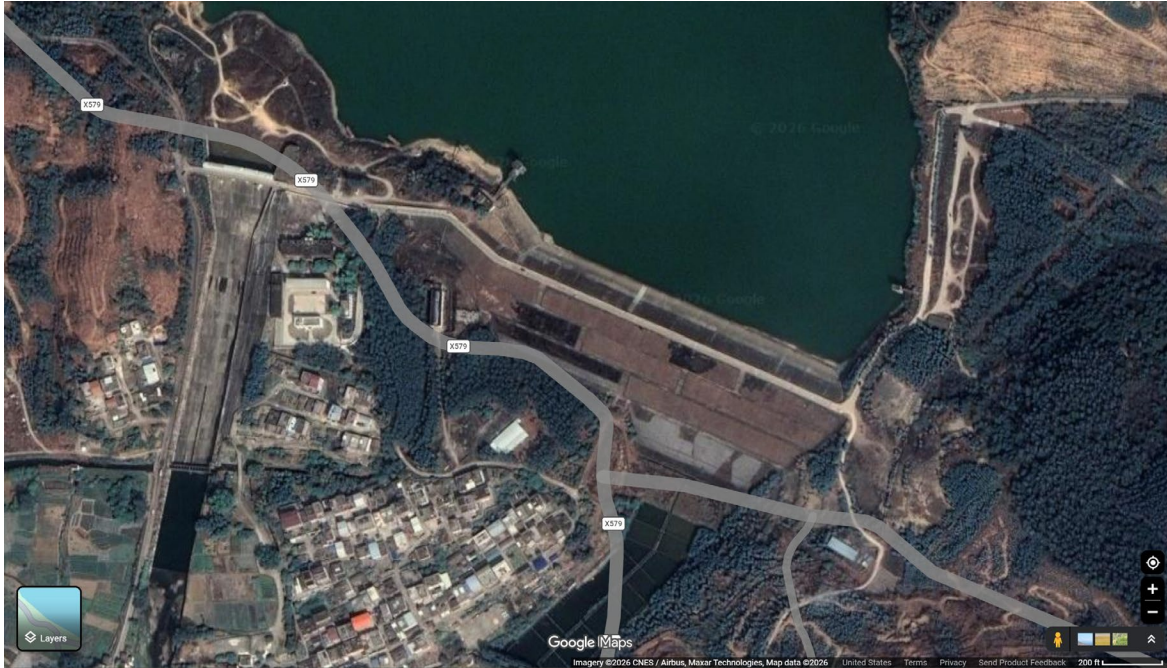
Figure 1. Pre-Event Layout of Liulan Reservoir and Satellite Image of the Channel Near the East Abutment. The open bypass-like channel outside the abutment is visible on the right. Public reporting has associated it with a fuse-plug emergency spillway, but its formal function, control elevation, and relationship to the initial breach remain to be confirmed from design records and the investigation. Image source: Google Maps (imagery credits shown in the figure).
