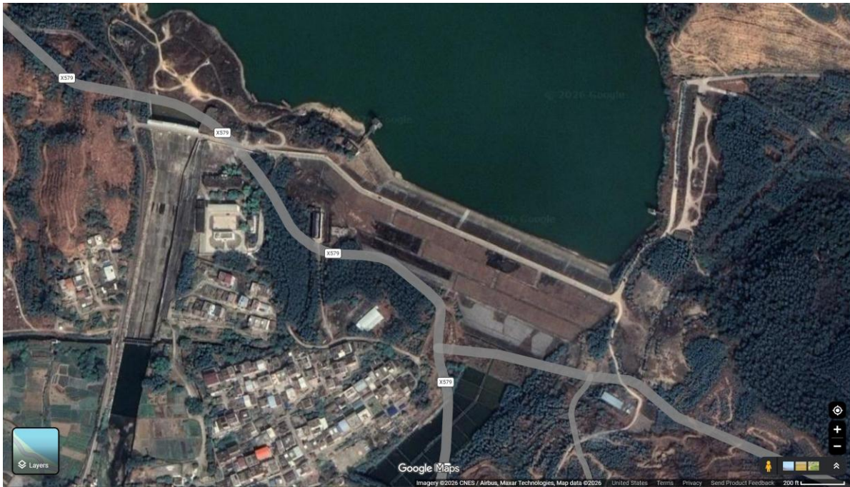
Figure: Pre-event satellite imagery of Liulan Reservoir engineering layout (Google Maps; imagery source: Imagery ©2026 CNES / Airbus, Maxar Technologies)
